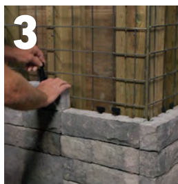
3 Attach Tandem Veneer with Connector
