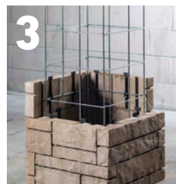
3 Repeat step 2 and fill with ¾" crushed rock until column is complete
